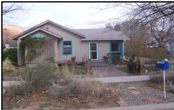
The above home is a good example of breaking up wall length and height with variations in roof line and footprint.
