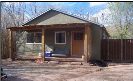
The above home is an example of breaking up wall height with the addition of a porch.
