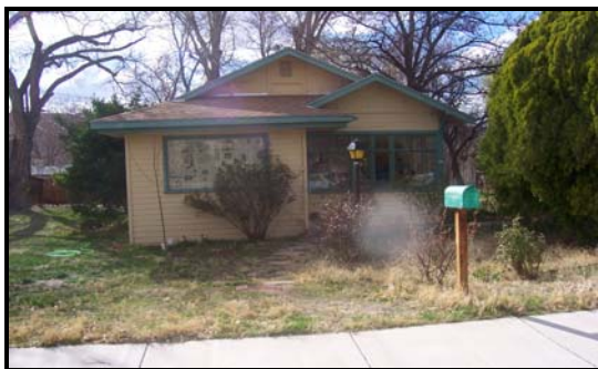
The above home is a good example of breaking up wall length and height with variations in roof line.
