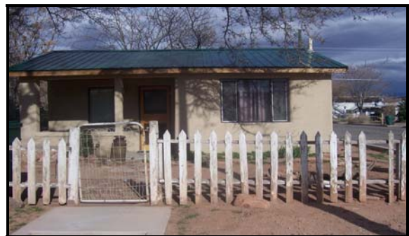
The above home is a good example of breaking up wall length with a recessed porch.
