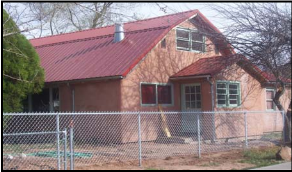
The above home is a good example of breaking up a back wall with the addition of a bump out.
