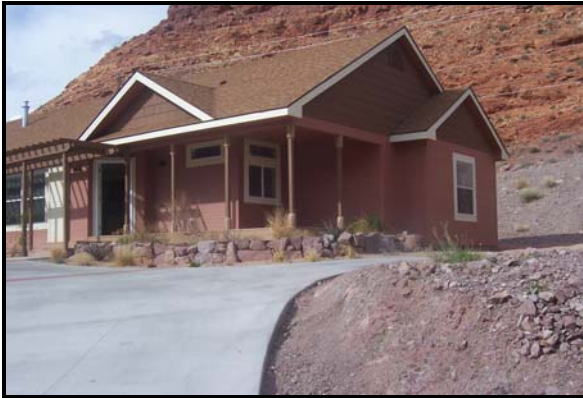
The above home is a good example of breaking up long walls with the recessed porch and the bump out on the side.
